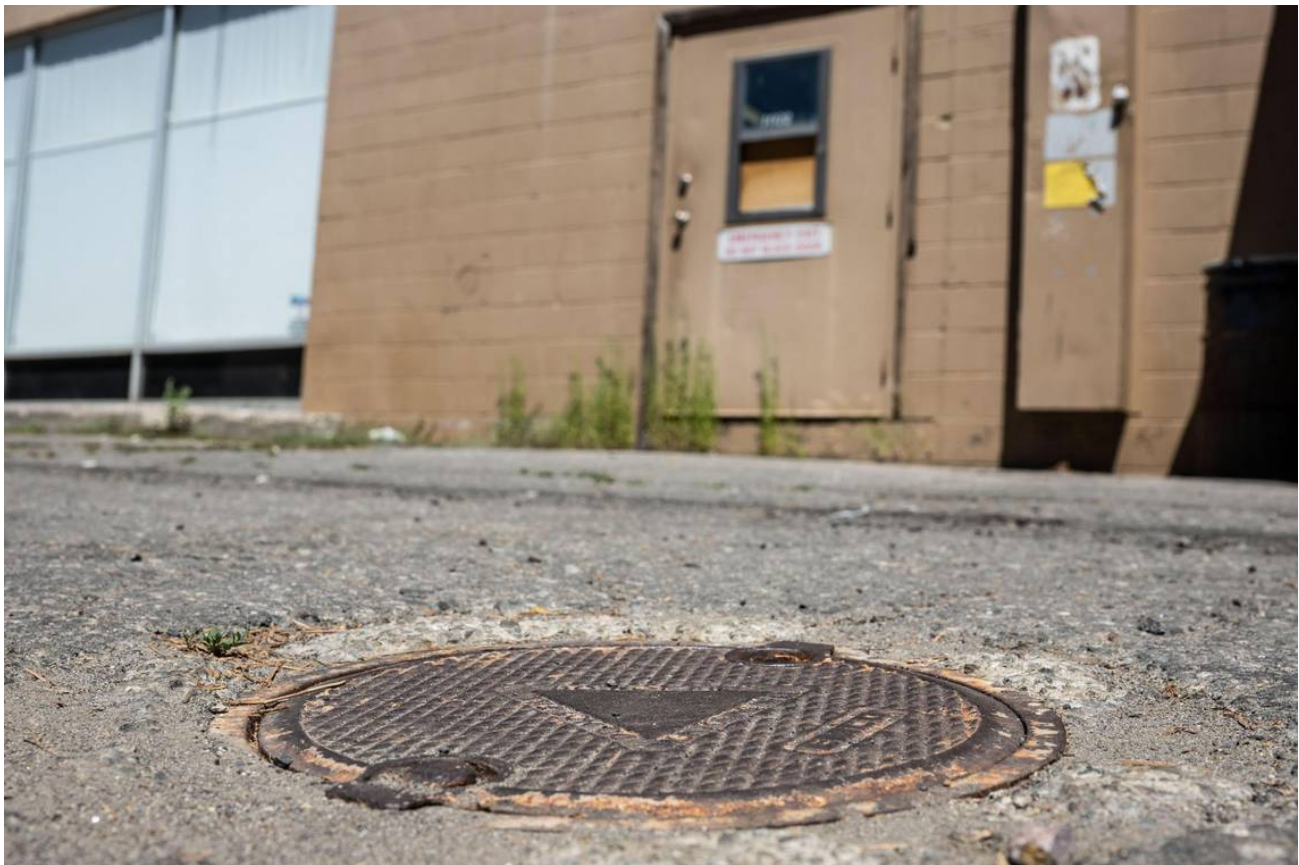
A maintenance hole for a groundwater monitoring well at the site of a former dry cleaning business in South Lake Tahoe. Hector Amezcua hamezcua@sacbee.com
